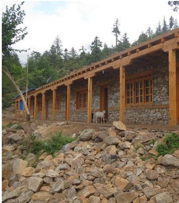
The nearly finished new house
