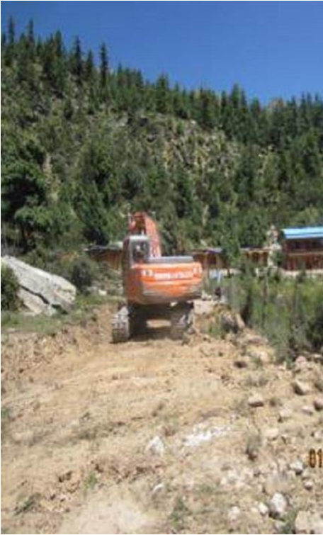
The road is being built to the school home.
