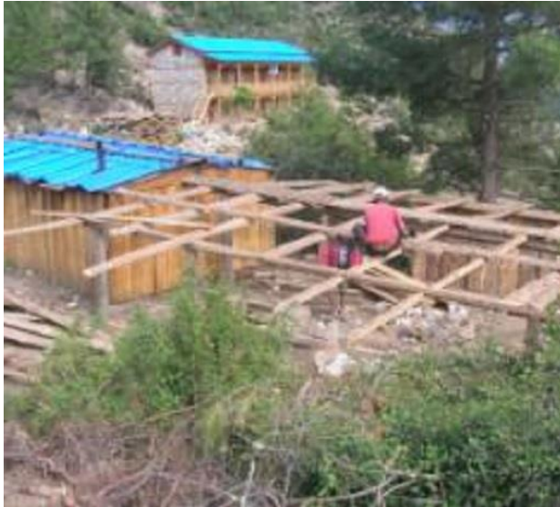
The dining hall under construction
