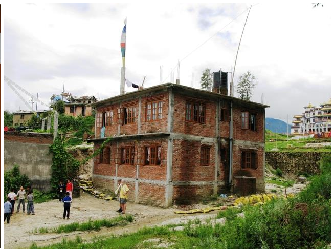
KMCH rented the first floor in this house
