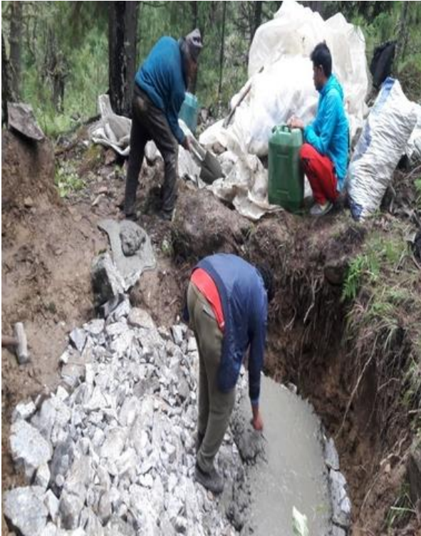
Work with the new waterpipes. All is done by hand.
