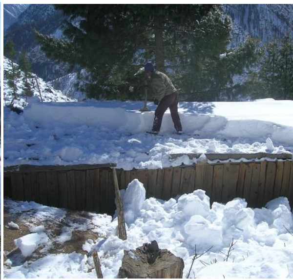
The snow is taken away from the roof of our kitchen
